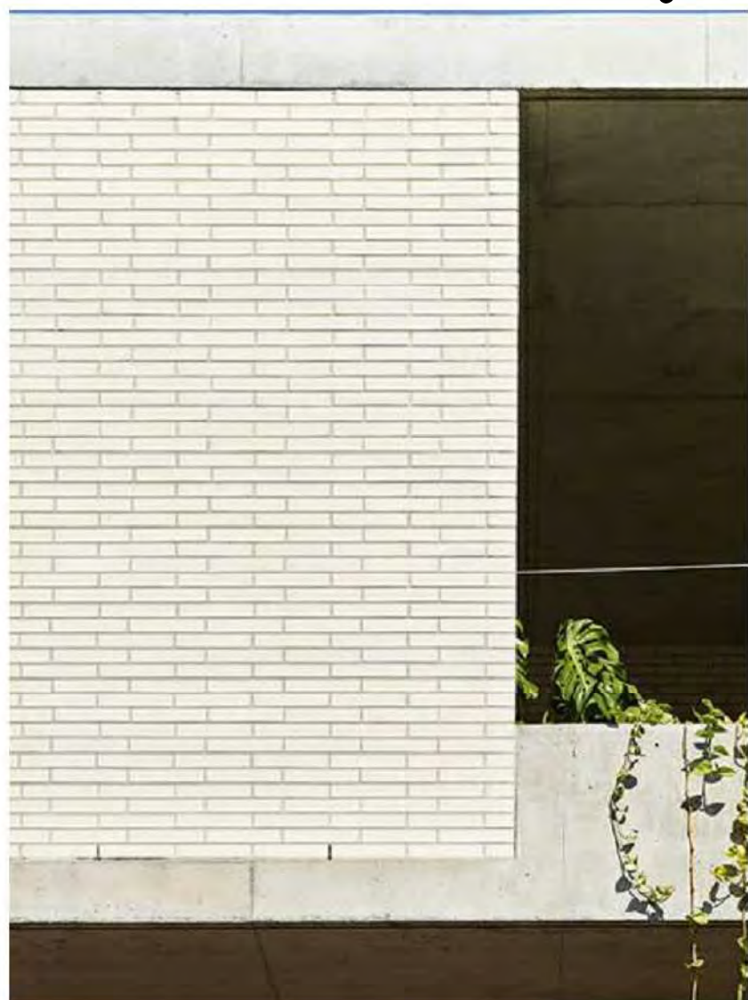
WHITE BRICK & CONCRETE
