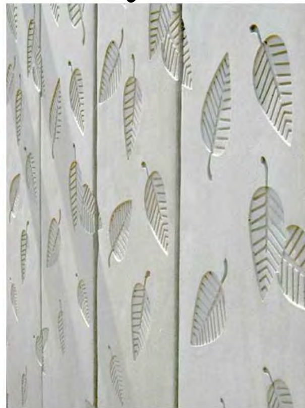
CONCRETE PRECAST PANEL WITH LEAF MOTIF
